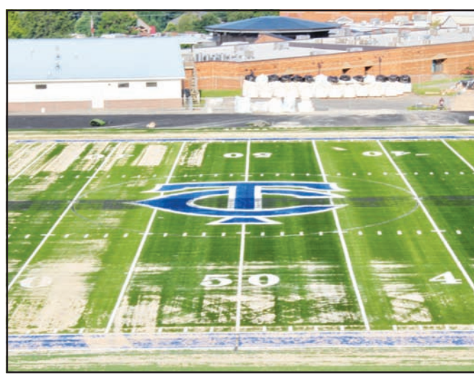
A view of the new artificial turf field at Towns County High just prior to the final brushing of sand and rubber inlay over the weekend. Photo by Chad Stack
